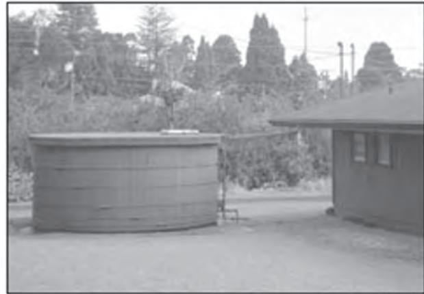
Figure 1. Harvesting rainwater, a recommendation for the sustainable management and best use of water in buildings (source: Center for Maximum Potential Building Systems, Texas Guide for Rainwater Harvesting, TWDB, Texas Center, Texas, 1995).
