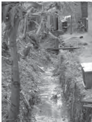
Side ground ditches dug by water during their flow, and of... ground drains worked out by the inhabitants. ©Nguendo Yongsi, 2006
