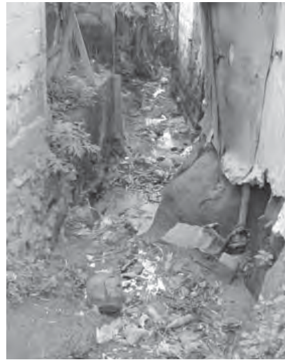
Figure 5. Open gutters blocked by household refuse and covered with vegetation in Yaoundé
